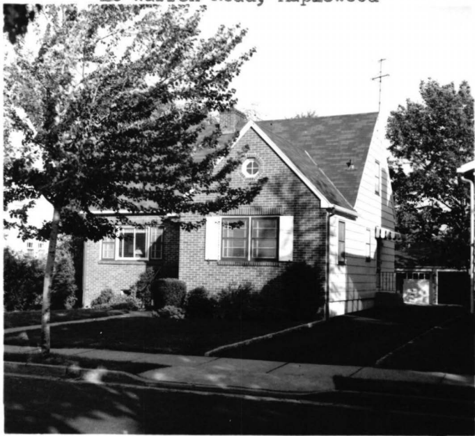
10 Warren Road, Maplewood
